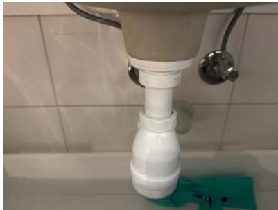
Røropplegg under servant.
