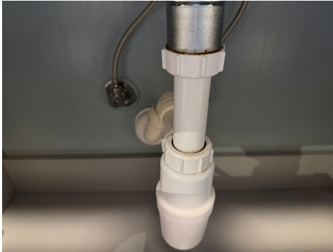
Røropplegg under servant.
