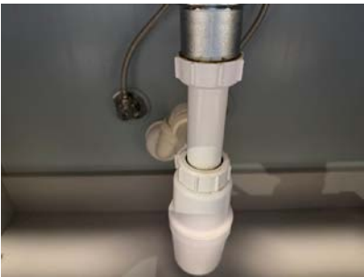
Røropplegg under servant.
