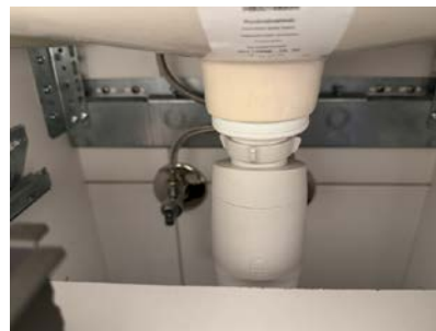
Røropplegg under servant.
