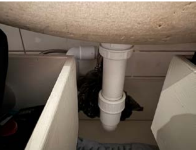
Røropplegg under servant.
