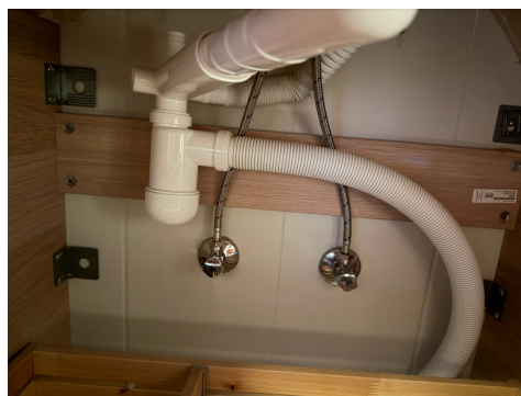
Røropplegg under servant.
