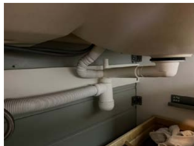
Røropplegg under servant.
