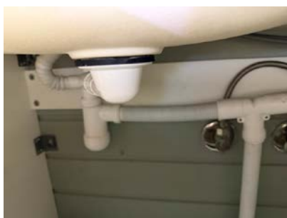
Røropplegg under servant.
