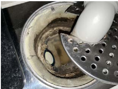
Sluk under servant.
