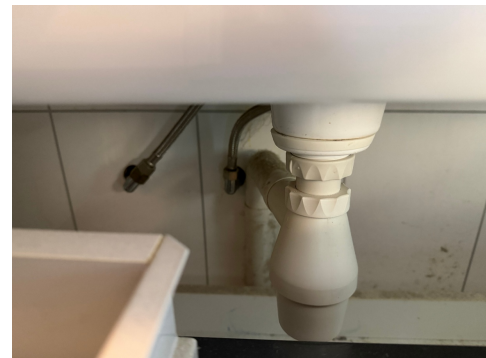
Røropplegg under servant.
