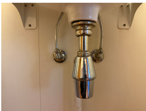
Røropplegg under servant.
