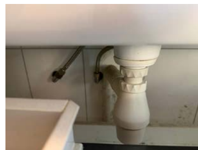
Røropplegg under servant.
