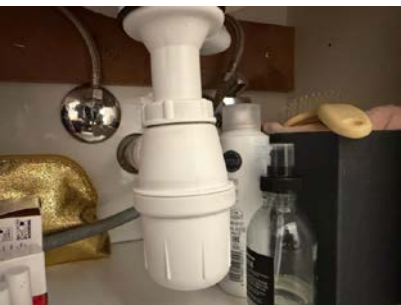
Røropplegg under servant.
