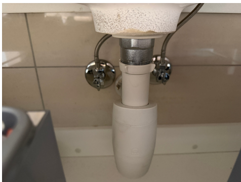
Røropplegg under servant.
