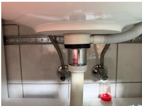
Røropplegg under servant.
