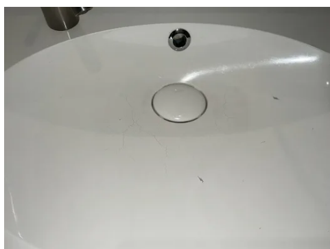
Krakelering i servant.
