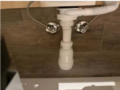
Røropplegg under servant.
