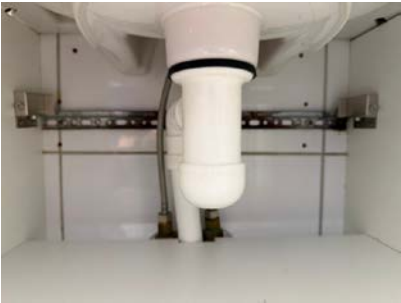
Røropplegg under servant.
