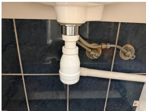
Røropplegg under servant.
