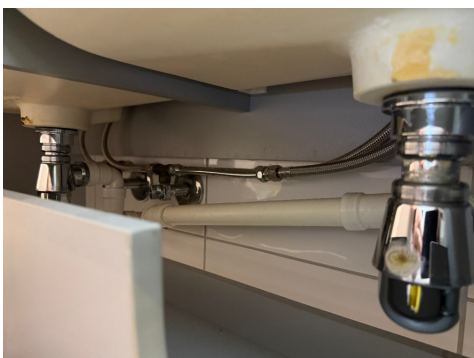
Røropplegg under servant.
